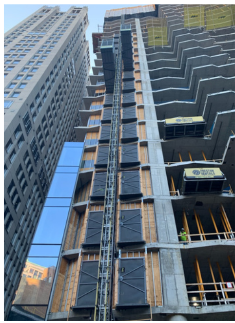
CONEY ISLAND, NY - MAST CLIMBERS, SUSPENDED AND SUPPORTED SCAFFOLD, AND HOIST SYSTEM
