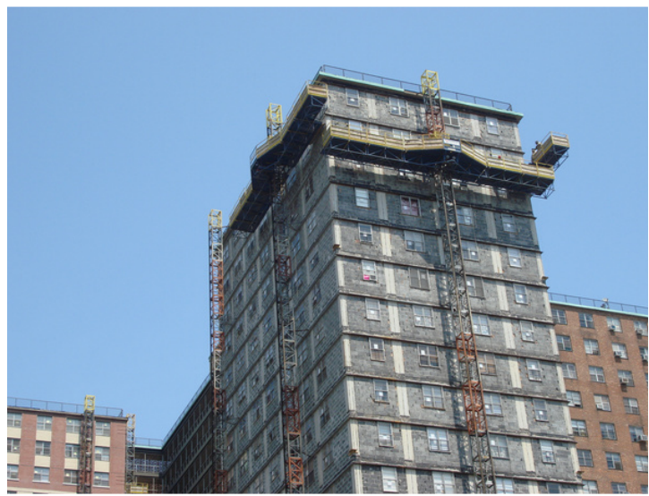
CONEY ISLAND, NY - MAST CLIMBERS, SUSPENDED AND SUPPORTED SCAFFOLD, AND HOIST SYSTEM
