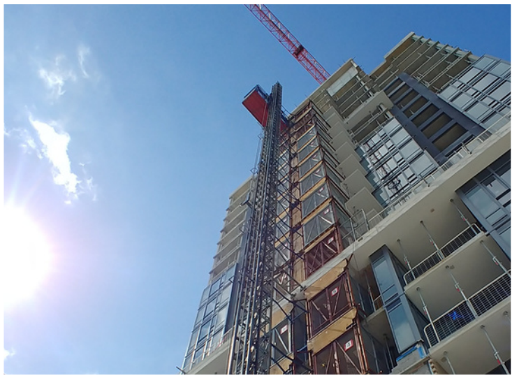
CITIZEN M, MIAMI, FL - DUAL CONSTRUCTION HOIST (1 UNIT)
