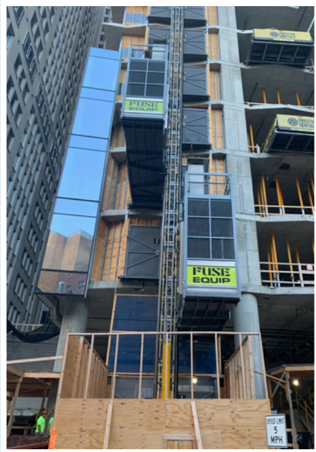
CONEY ISLAND, NY - MAST CLIMBERS, SUSPENDED AND SUPPORTED SCAFFOLD, AND HOIST SYSTEM
