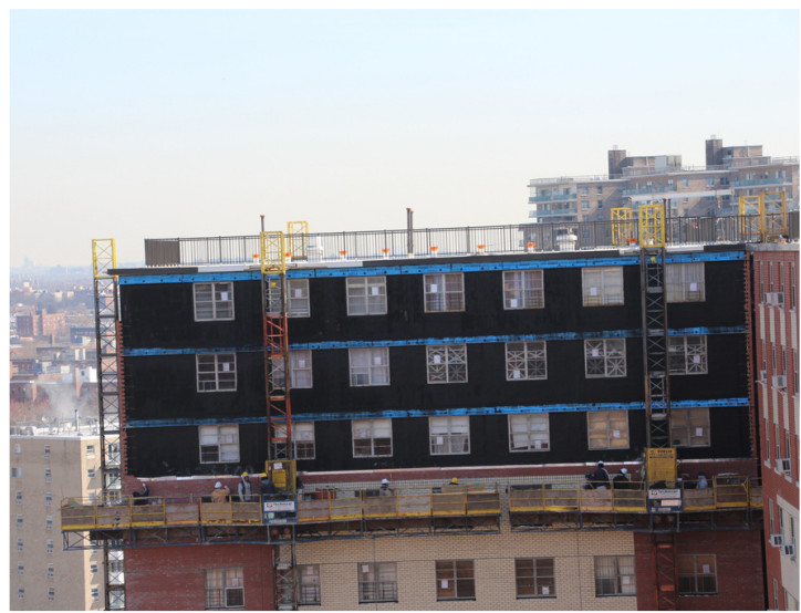
CONEY ISLAND, NY - MAST CLIMBERS, SUSPENDED AND SUPPORTED SCAFFOLD, AND HOIST SYSTEM
