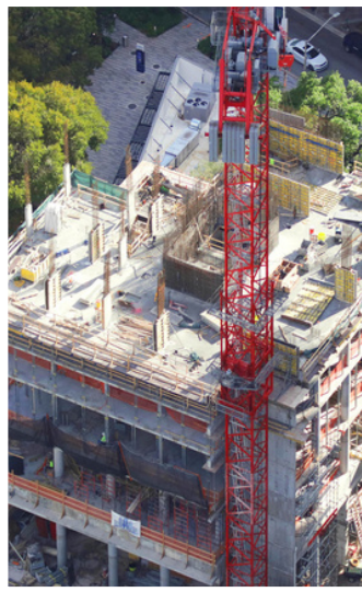
CITIZEN M, MIAMI, FL - DUAL CONSTRUCTION HOIST (1 UNIT)
